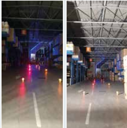
Storage hall illumination with an Energyline large-area floodlight. Left image: Floodlight switched off. Right image: Floodlight switched on.
